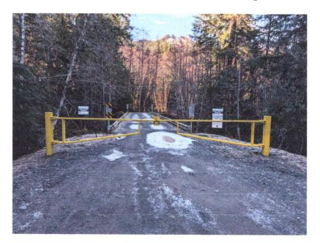
The above photo shows the new gate at Huckleberry Creek, which will be closed in the winter for habitat and elk protection. This gate, along with the gate at the upper 72 Road, is a welcome addition. That being said, it has a flaw: the space where the tongue can be accessed by a simple hacksaw and the fact that the piece is pot metal.
