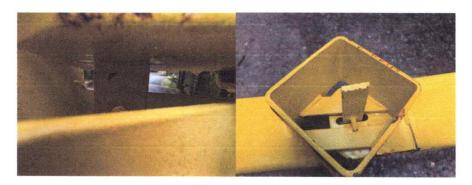
The photos above show these two problems. We suggest stainless steel for the drop pin in the right picture and a barrier welded to the side that will keep a hacksaw from accessing the side of the pin. In its current state, a hacksaw could cut the gate open in a few minutes or less. Stainless would give it a fighting chance, but a barrier would help even more.
